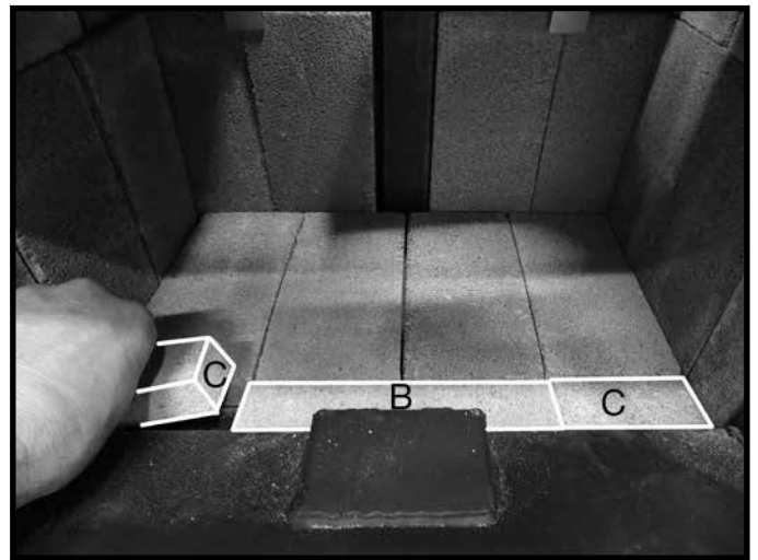
Figure 19: Narrow front bricks in place.
