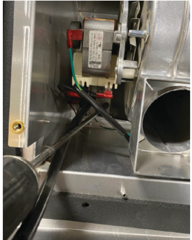
Figure 8.9 - Vacuum Switch Removal
