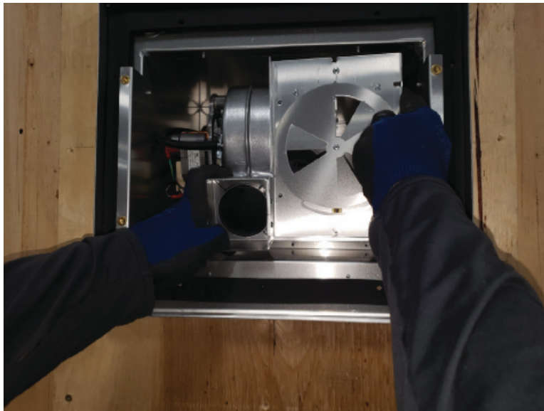
Figure 8.3 - Exhaust Assembly Removal
