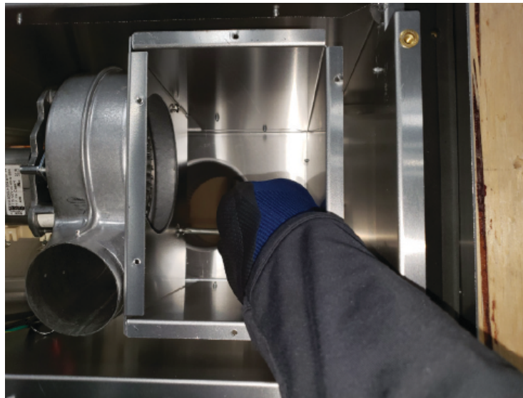
Figure 8.6 - Remove (3) Screws Securing Fan Assembly
