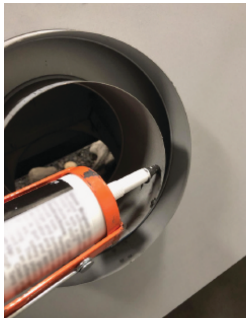
Figure 6.10 - Sealant on Inner Exhaust on Fireplace
