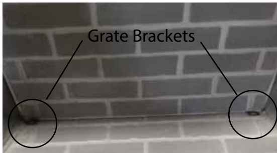
Figure 7.2 Grate Brackets In Place
