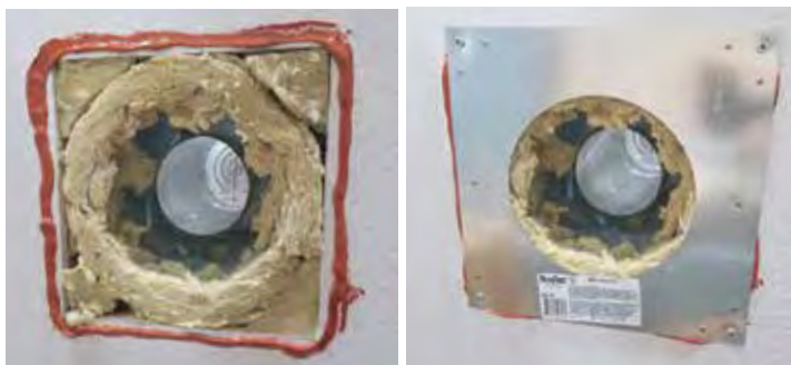
Figure 63: Thimble Insulation
