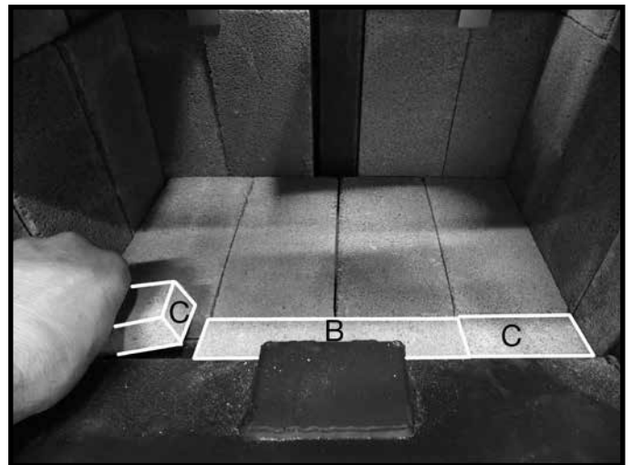
Figure 19: Narrow front bricks in place.
