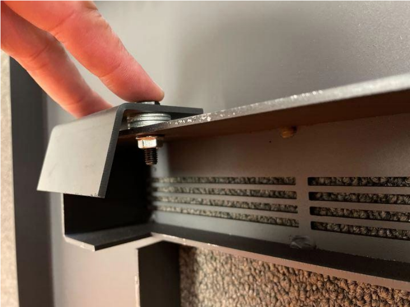
Attach surround hangers to the surround above the louvers, with hooks facing the bottom of the piece, and washers located as shown.
