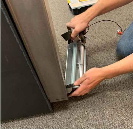
Slide blower assembly into side blower duct piece
