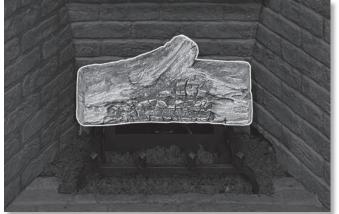
Figure 34: Log Set Installation - Step 1
