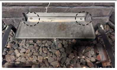
Figure 5: Venturi Cover Box Removal
