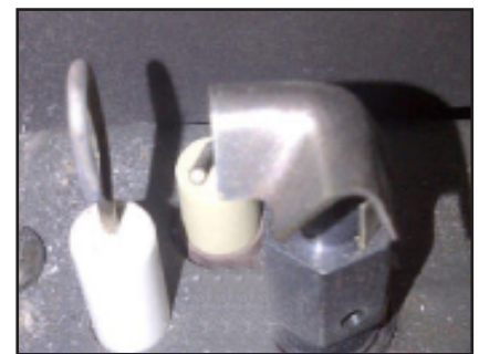
Figure 24: Proper Pilot Position
