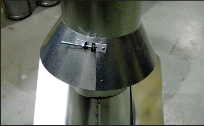
Figure 7.14 - Insert Bolt into Brackets
