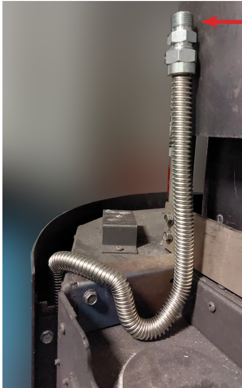
Figure 13: Flex Line Installation - Step 1
