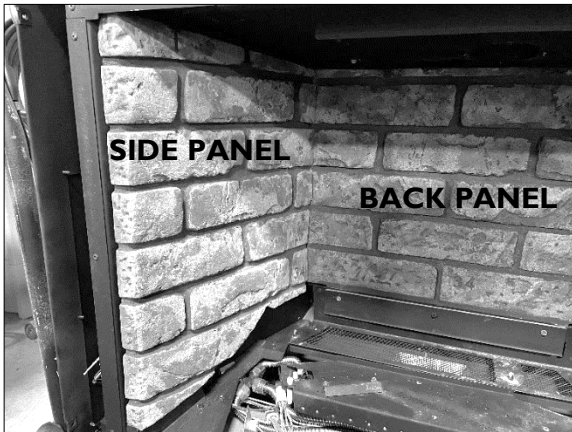
Figure 9.2, Refractory Panel Installation
