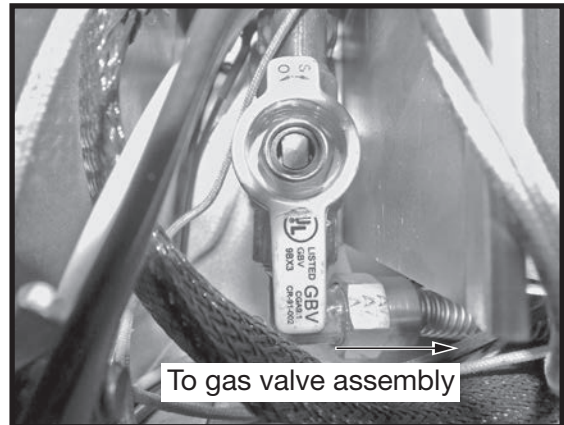
Figure 37: Gas shut off valve.
