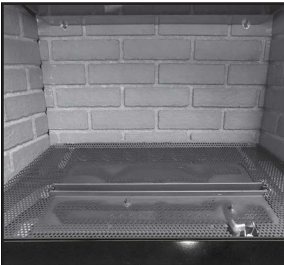
Figure 53: Burner with empty burner tray.
