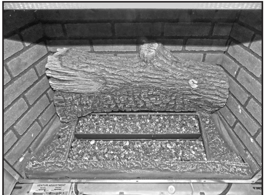
Figure 78: Ember pieces spread on top of burner trays.
