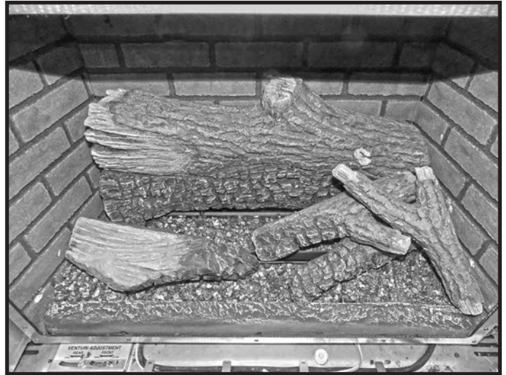
Figure 84: 5th log placement.
