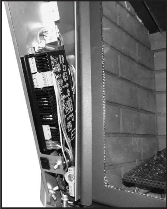
Figure 38: SIT control center.
