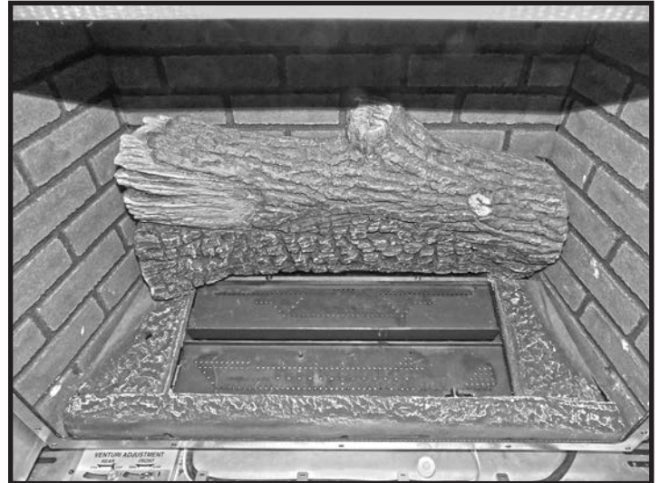
Figure 76: 1st log placement.
