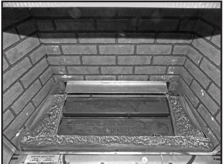
Figure 74: All three base pieces in place.
