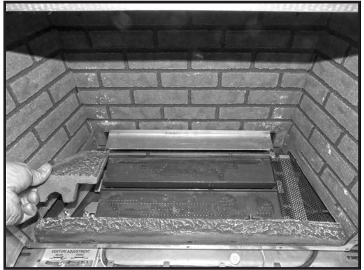
Figure 72: Installing left side base piece.
