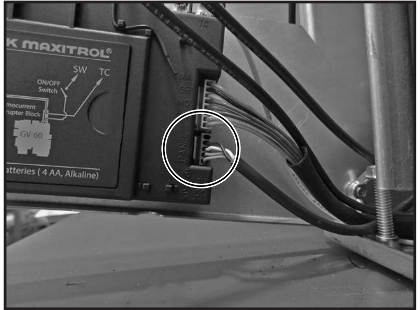
Figure 90: Switch connector at control module.
