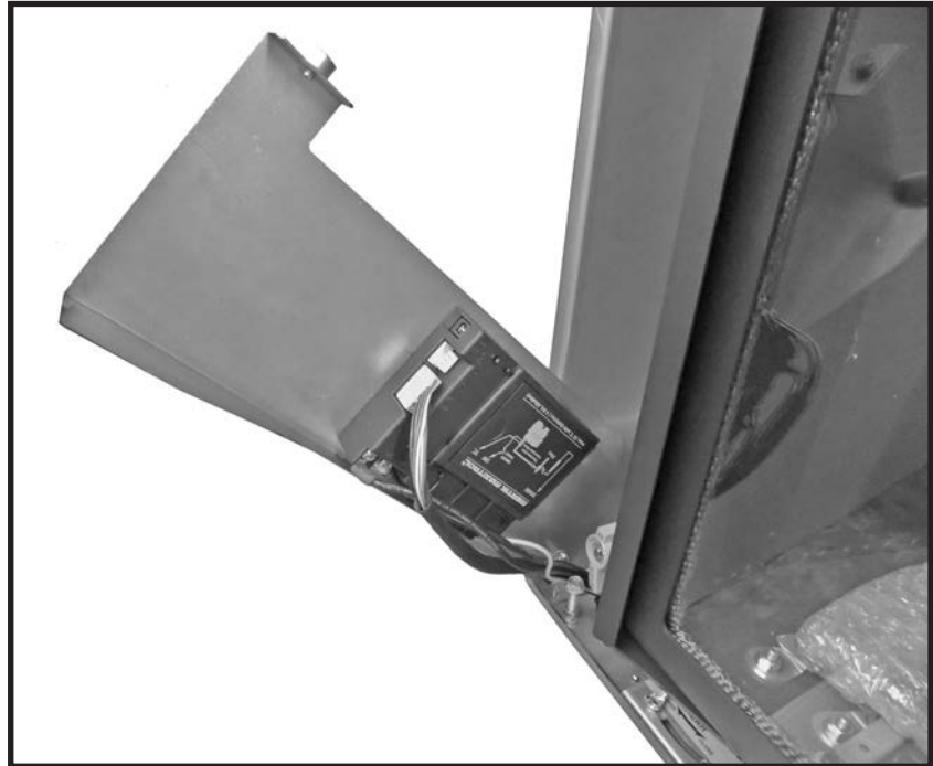
Figure 40: Maxitrol electrical controller in its caddy.
