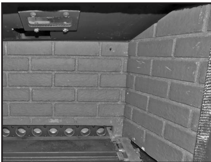
Figure 28: Right side panel in place.
