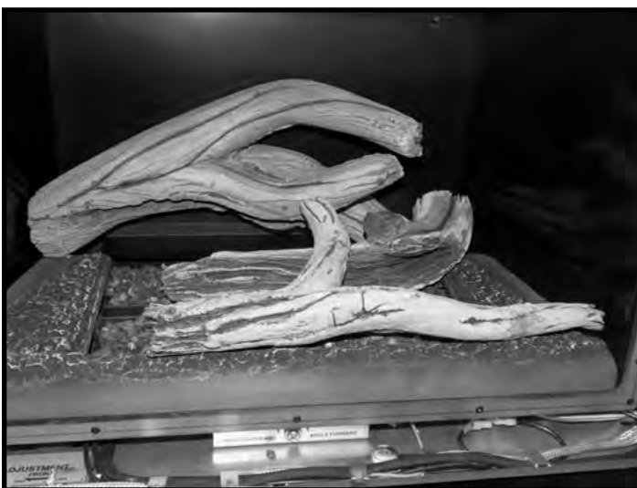
Figure 100: Third log placement .
