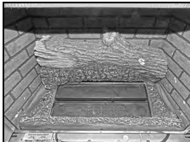
Figure 76: 1st log placement.
