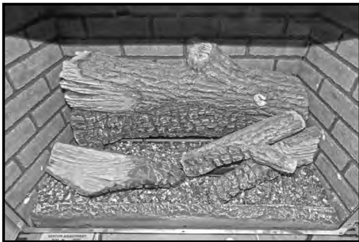
Figure 83: 4th log placement.
