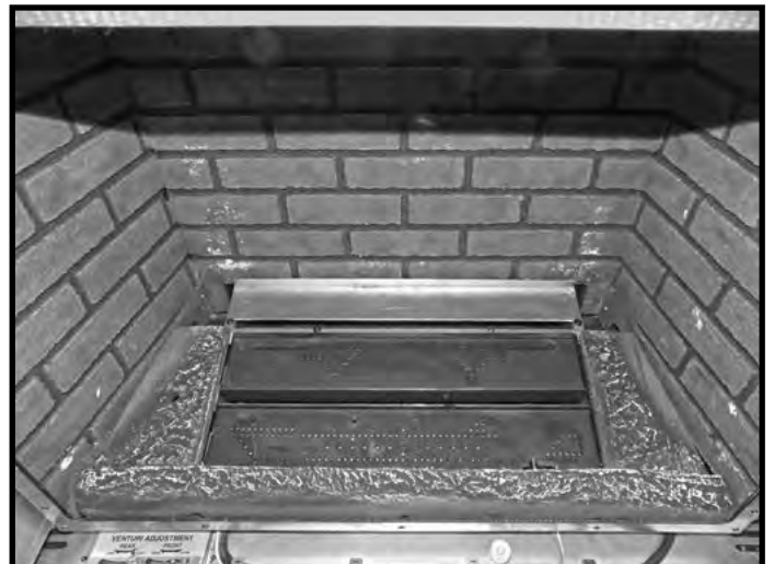
Figure 74: All three base pieces in place.
