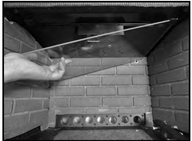
Figure 31: Inserting baffle into the upper corner.
