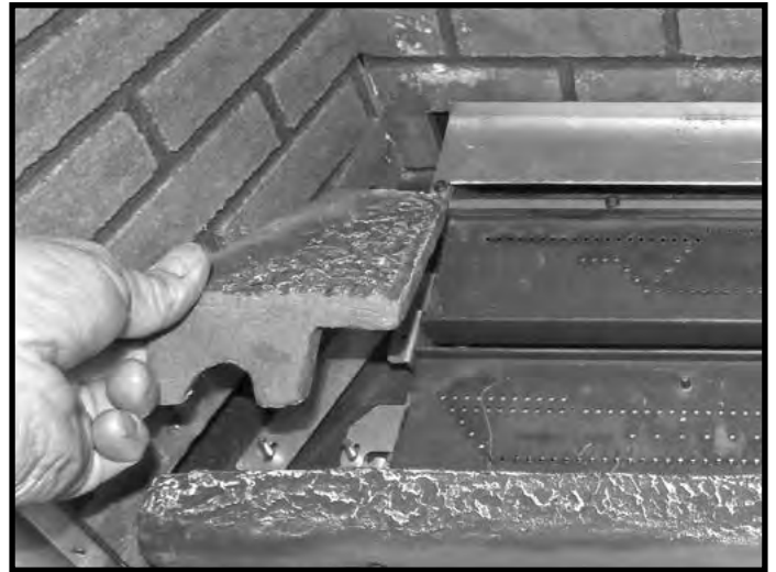
Figure 72: Installing left side base piece.
