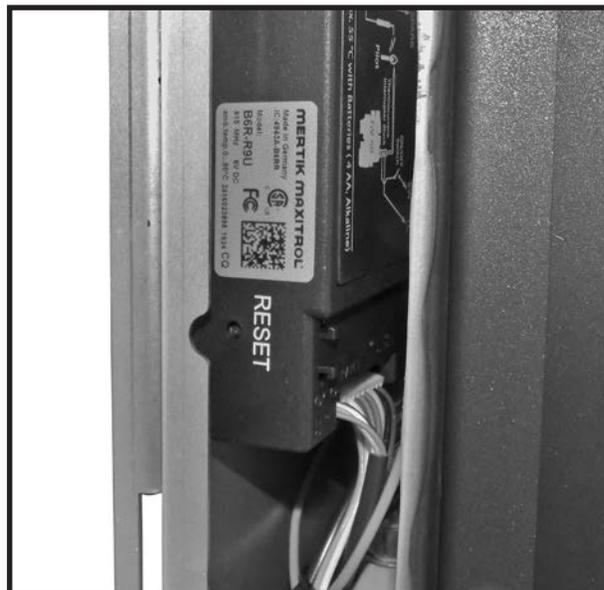
Figure 101: Maxitrol reset button location.
