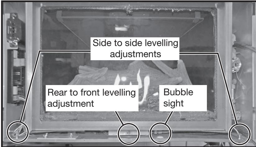
Figure 6: Leveling adjustments.
