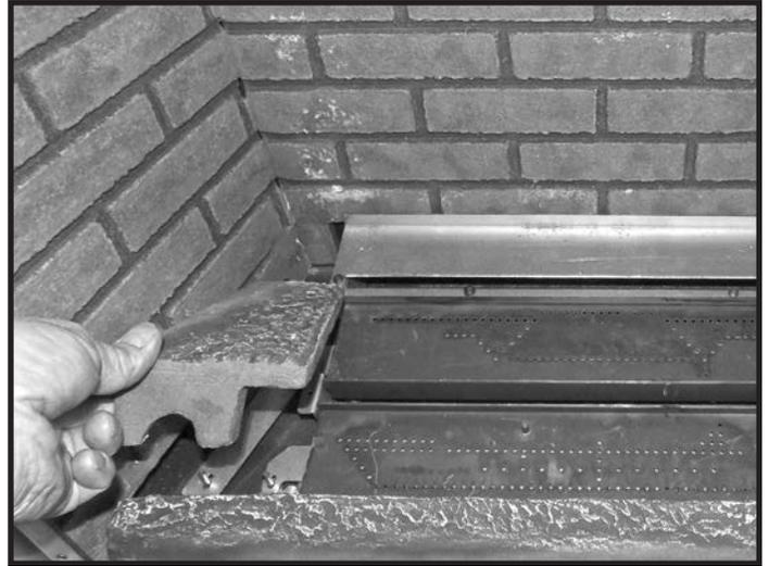
Figure 72: Installing left side base piece.
