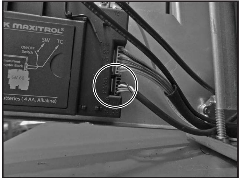
Figure 92: Switch connector at control module.
