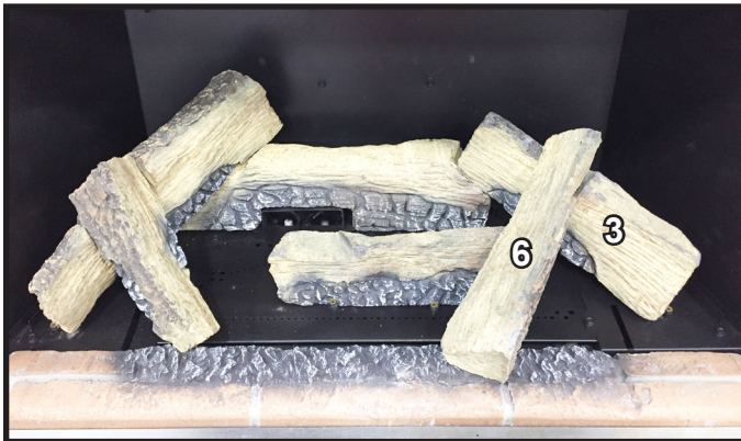
Figure 8. Log #6 Installed
