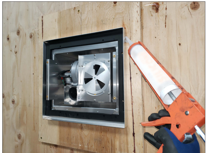
Figure 3.20, Silicone around the Cap Base
