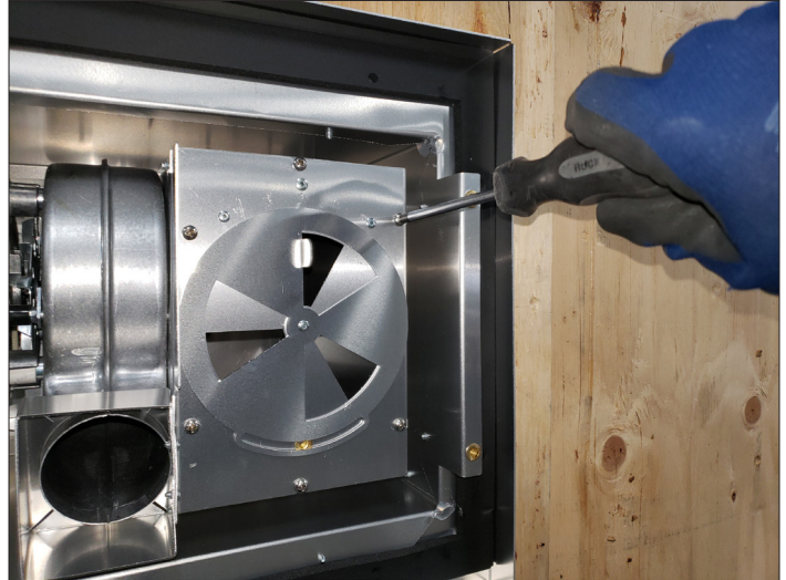
Figure 5.2, Exhaust Assembly Screws
