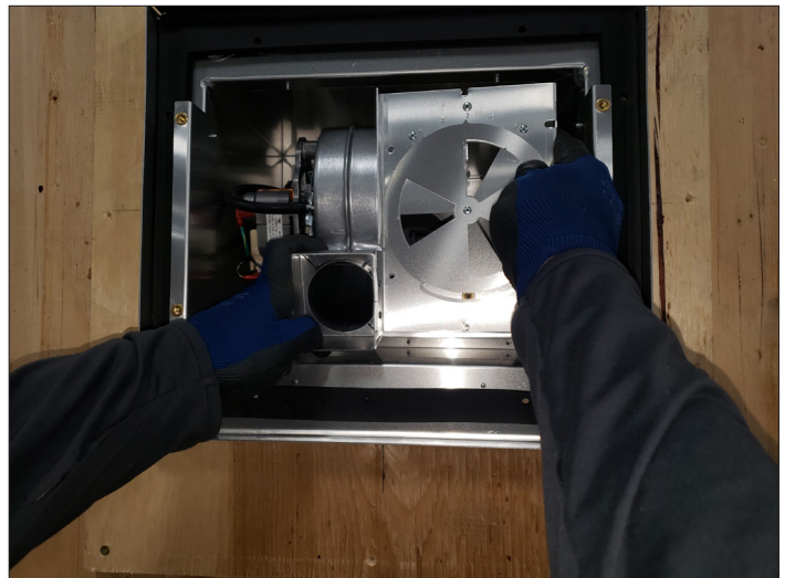
Figure 5.3, Exhaust Assembly Removal
