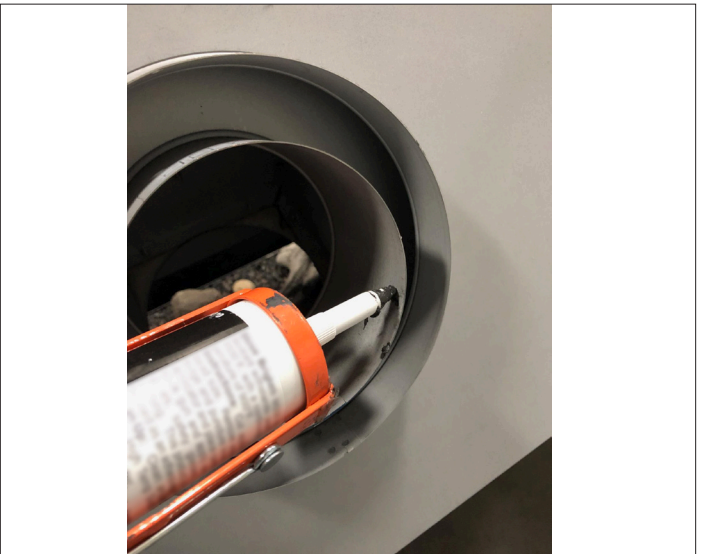
Figure 2.2, Apply Sealant to Inner Exhaust on Fireplace
