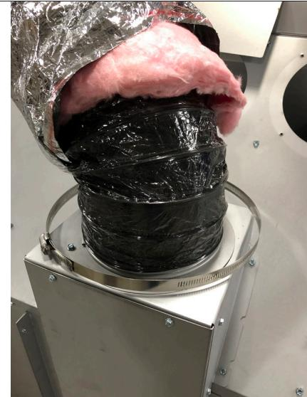
Figure 2.3, Band Clamp over HTK Air Chute Collar
