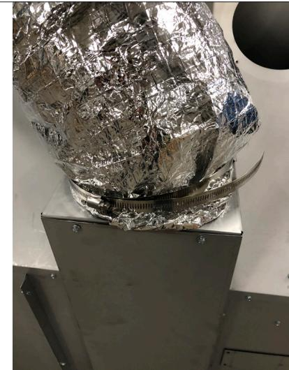
Figure 2.4, Band Clamp Securing Outer Insulation to Inner Pipe and Collar
