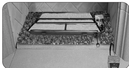
Fig. 17-3 Place sand (if applicable)
