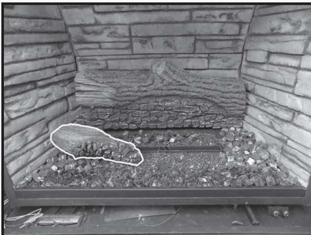
Figure 80: 2nd log in place.
