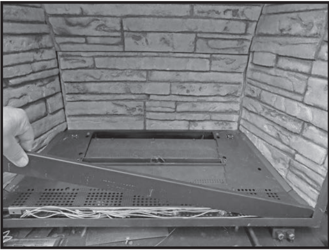
Figure 73: Covering wires with front trim piece.
