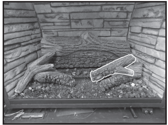
Figure 83: 5th log in place.
