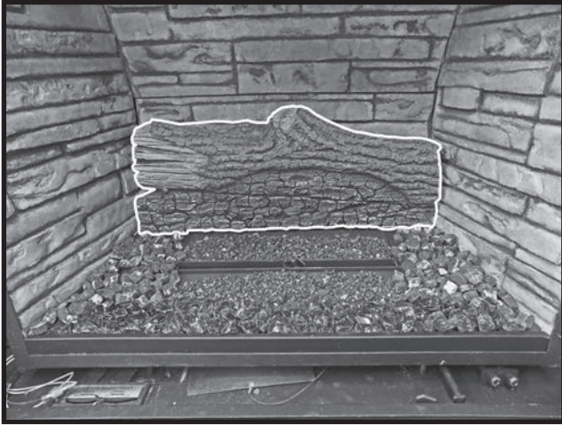
Figure 77: First log in place.
