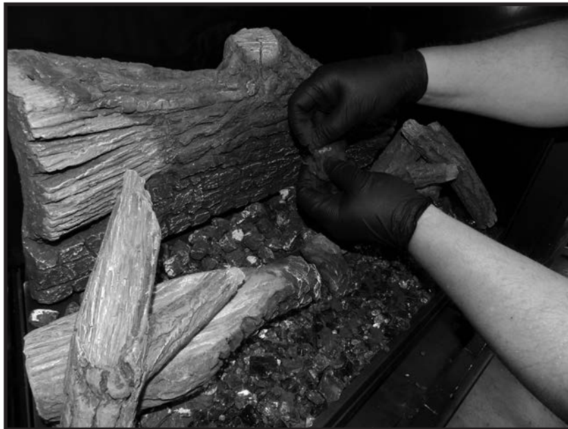
Figure 91: Applying ember wool blend in transition lines.
