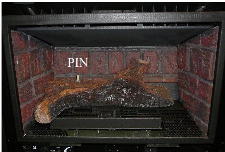
Figure 68. First Stage Log Set Installation.
