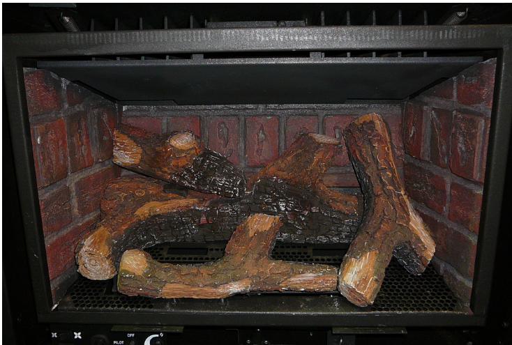
Figure 71. Fourth Stage Log Set Installation.
