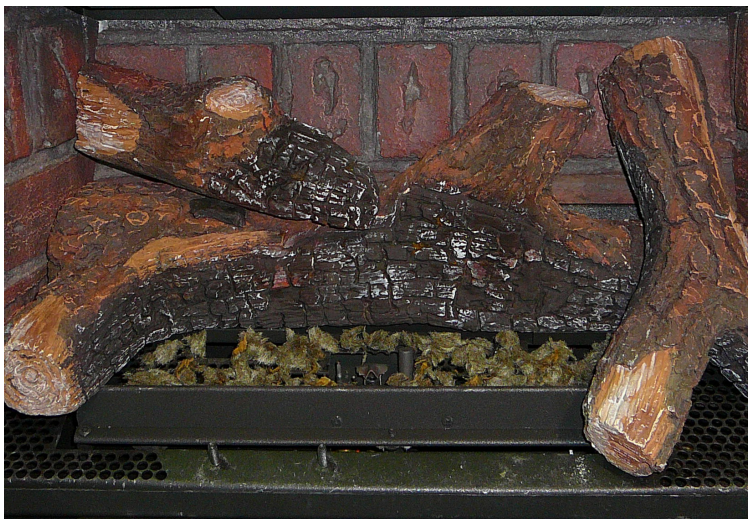
Figure 72. Fifth Stage Log Set Installation.
