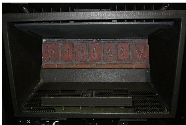
Figure 65: Back Brick Panel in Place.
