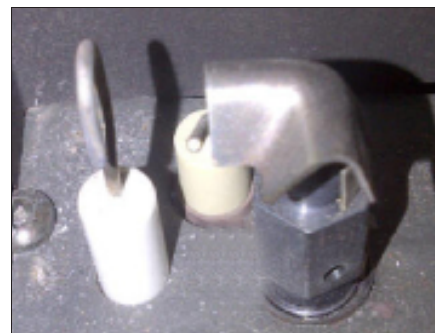
Figure 25 Proper Pilot Position
