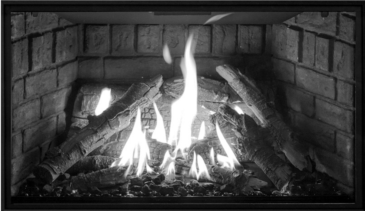
Figure 54. Proper Installation & Flame Appearance
