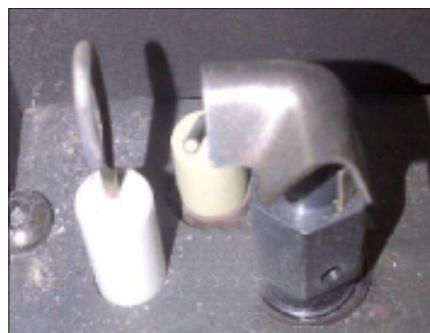
Figure 23 Proper Pilot Position
