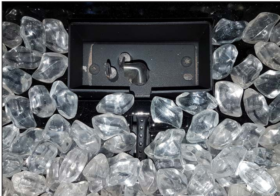
Figure 56: Correct glass media placement around pilot area
