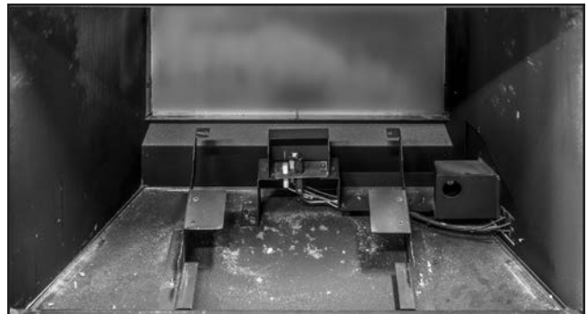
Figure 52: The rear liner can now be removed. Use a vacuum to clean up the bare firebox if needed.
