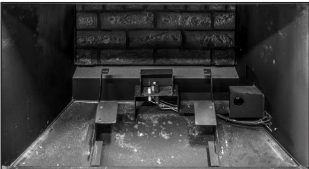
Figure 51: Lift the burner off the mounts and pull it out of the inlet box. The unscrew the panel brackets (T20's) from each side of the baffle to remove the left and right side liners.
