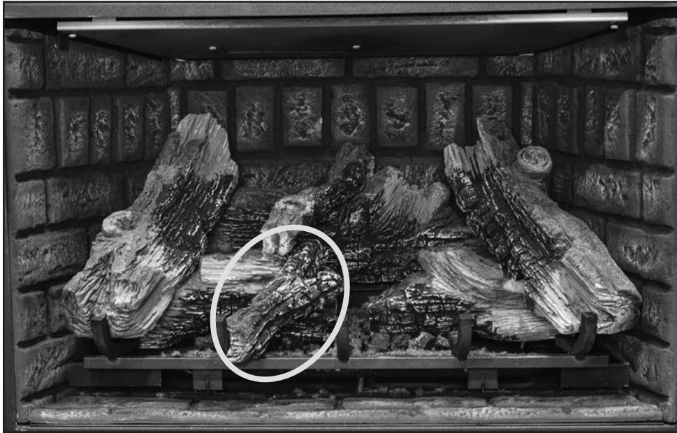
Figure 59: Rest the center top log on top of the left mid log making sure to align the bottom with grate arm.
