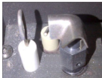
Figure 23 Proper Pilot Position
