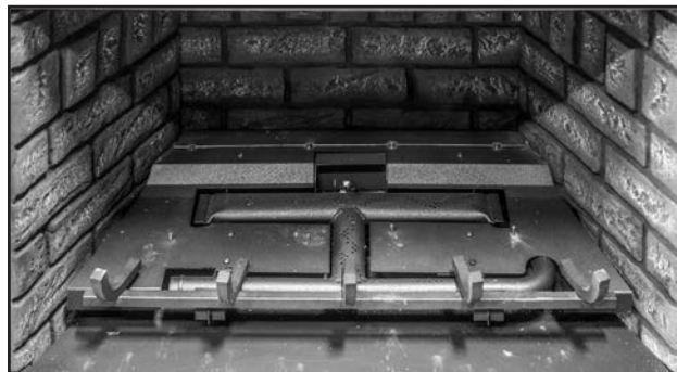
Figure 45: Carefully remove the front liner (if installed) on the bottom of the firebox by picking it up gently.
