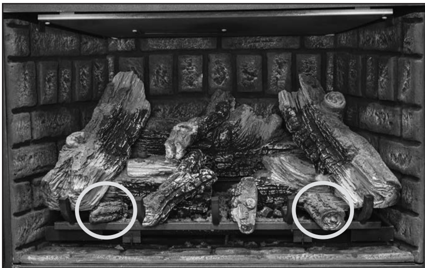
Figure 58: Finally, rest the left and right front chunks on the log grate and burner as shown.
