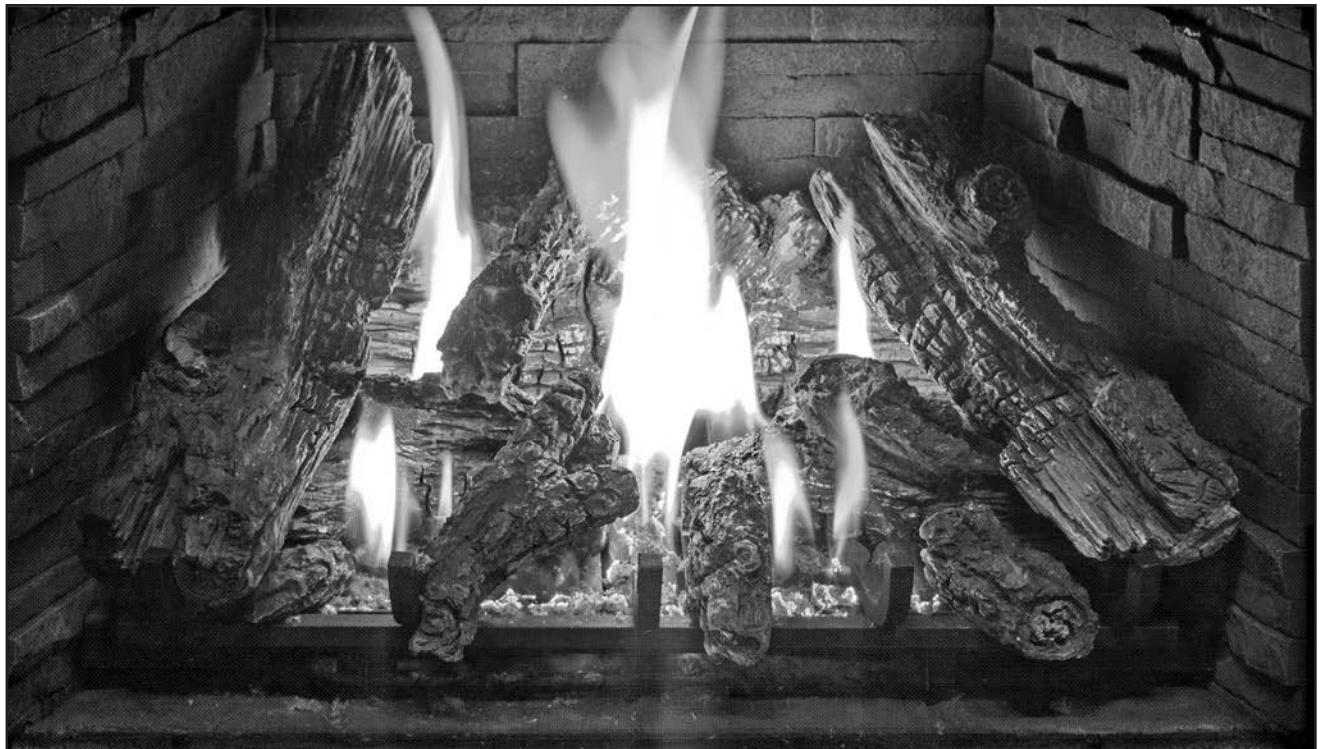
Figure 63: Proper installation and flame appearance
