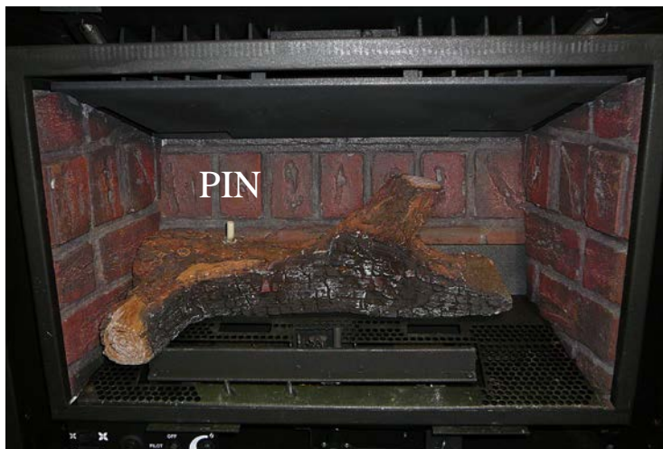
Figure 68. First Stage Log Set Installation.
