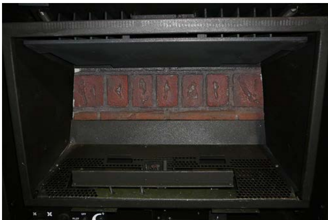
Figure 65: Back Brick Panel in Place.
