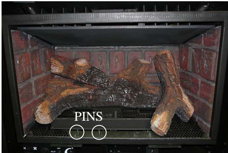
Figure 70. Third Stage Log Set Installation.
