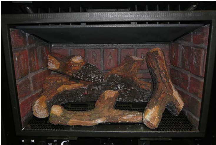
Figure 71. Fourth Stage Log Set Installation.
