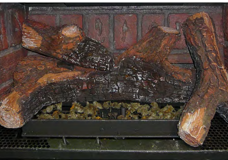
Figure 72. Fifth Stage Log Set Installation.
