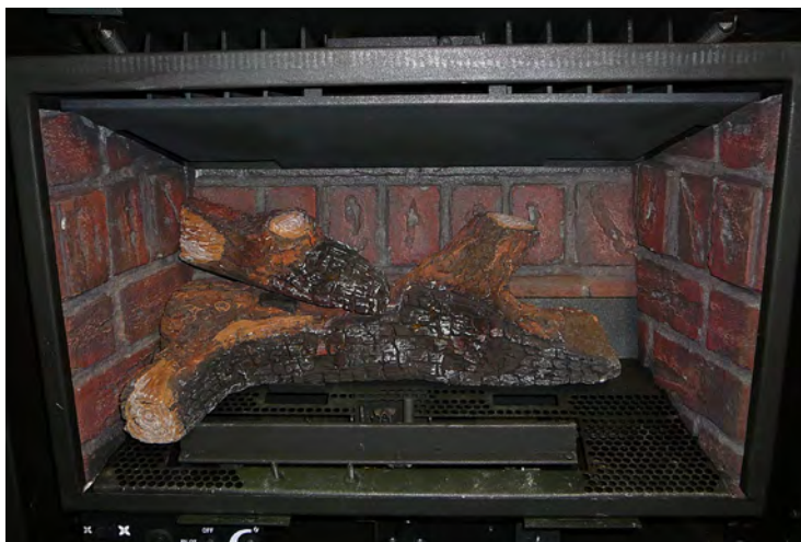
Figure 69. Second Stage Log Set Installation.
