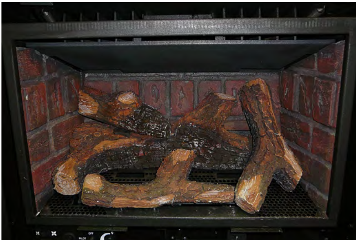
Figure 71. Fourth Stage Log Set Installation.
