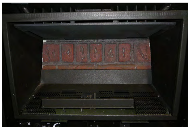
Figure 65: Back Brick Panel in Place.
