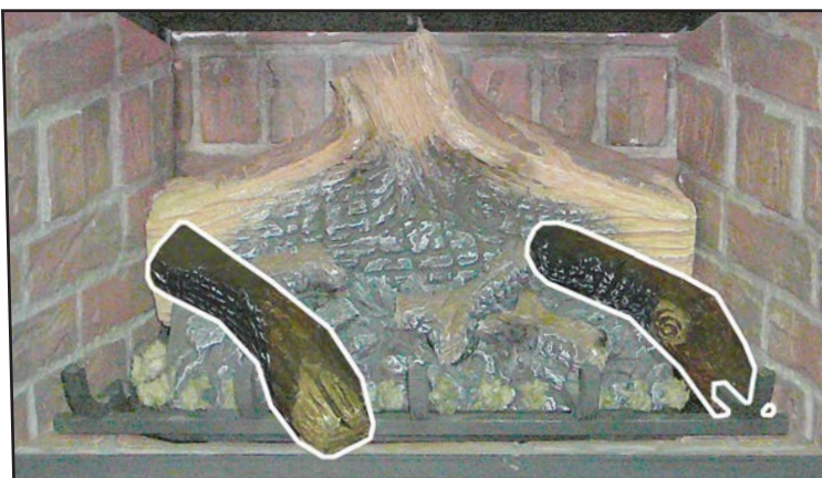
Figure 59: Fifth Stage Log Set Installation.
