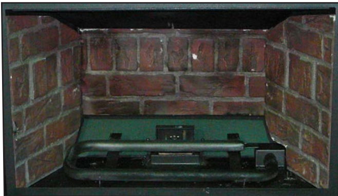
Figure 50: To remove the burner tube, gently pull it out of the venturi box.
