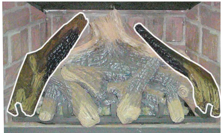
Figure 62: Eighth Stage Log Set Installation.
