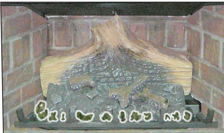
Figure 58: Fourth Stage Log Set Installation.
