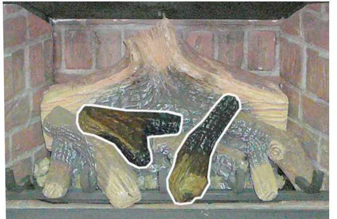
Figure 61: Seventh Stage Log Set Installation.
