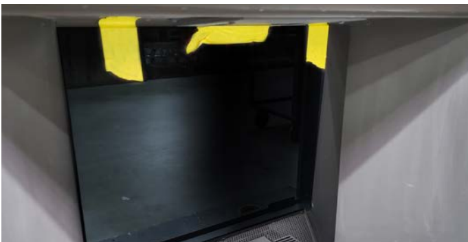
Figure 20.b hold it in place using masking tape
