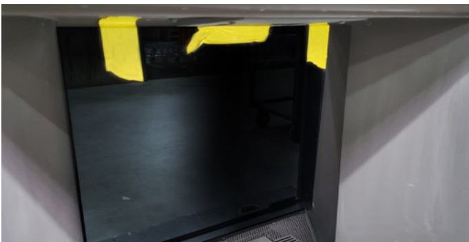
Figure 20.b hold it in place using masking tape
