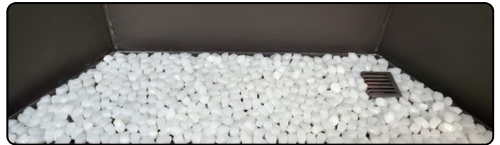
Figure 24.bb Completed firestone installation
