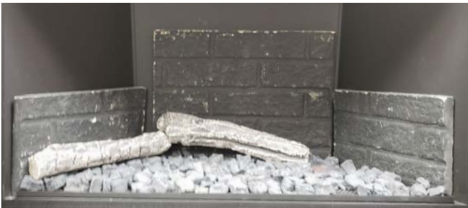
Step 3: Log B is placed in the right side of the firebox, resting the non forked end on log C
