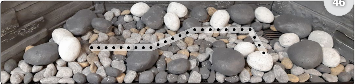
Figure 24.cc Completed Stone installation
