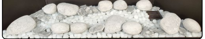
Figure 24.dd Completed ceramic chip installation
