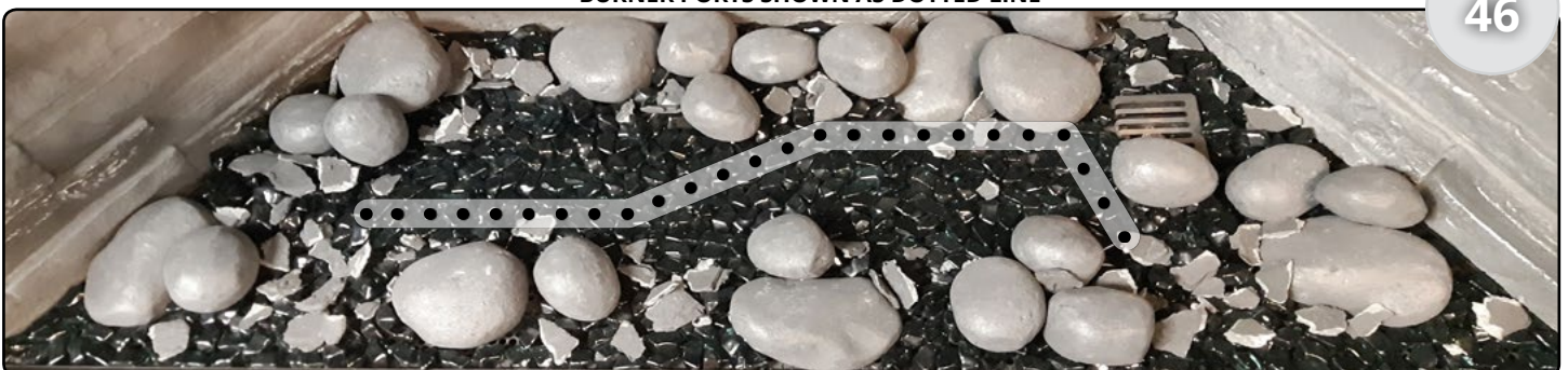
Figure 24.c Completed Stone installation
