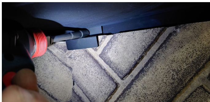
Figure 20.b Secure with the bracket using screw
