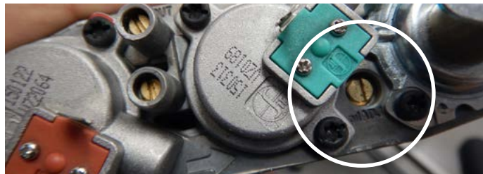
Figure 13.g Adjust pilot size
