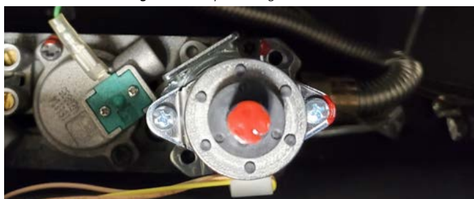
Figure 13.eee LP pressure regulator on a Full Load
