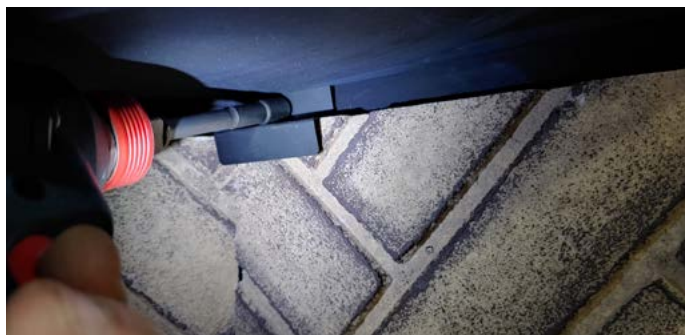
Figure 20.b Secure with the bracket using screw
