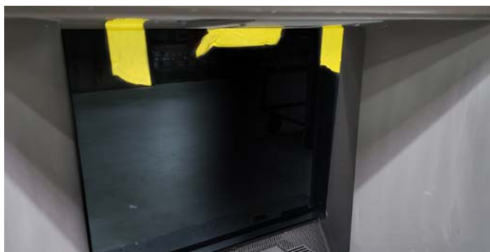
Figure 20.b hold it in place using masking tape
