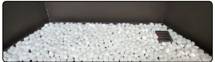
Figure 24.bb Completed firestone installation
