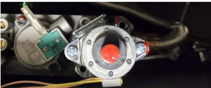
Figure 13.eee LP pressure regulator on a Full Load
