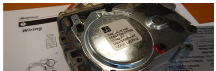
Figure 13.k Conversion label on valve
