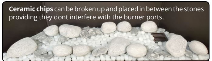
Figure 24.dd Completed ceramic chip installation
