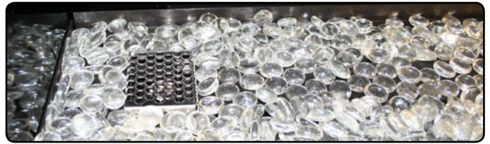
Figure 24.b Completed firestone installation
