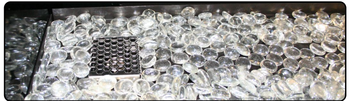
Figure 24.b Completed firestone installation
