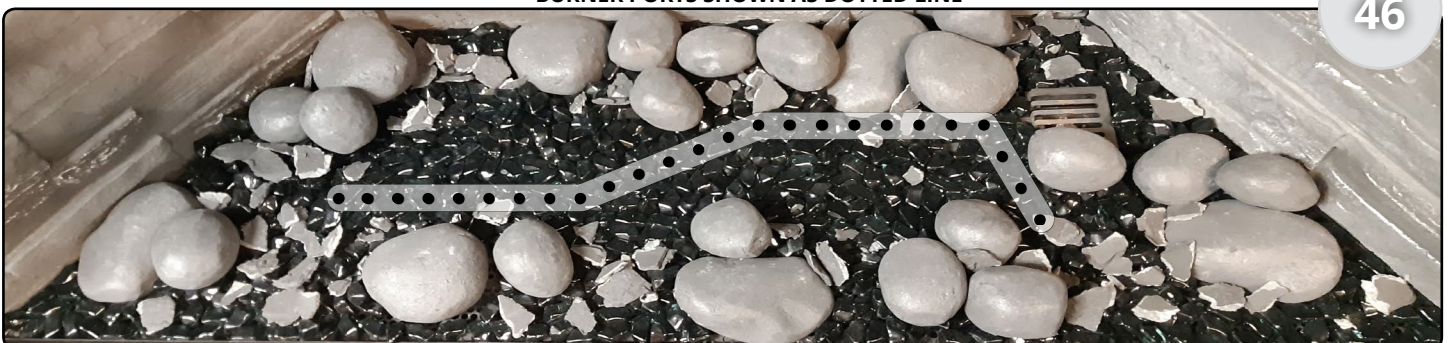
Figure 24.c Completed Stone installation
