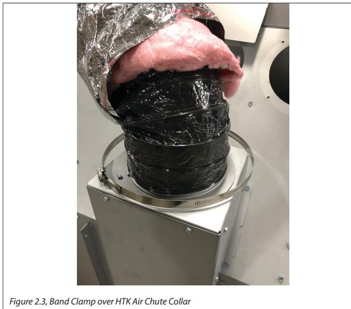
Figure 2.3, Band Clamp over HTK Air Chute Collar
