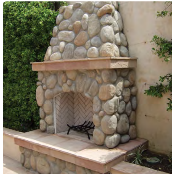
Contractor's Model Fireplace with stone veneer
