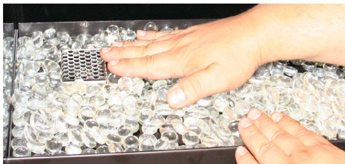
Figure 14b Completed firestone installation.
