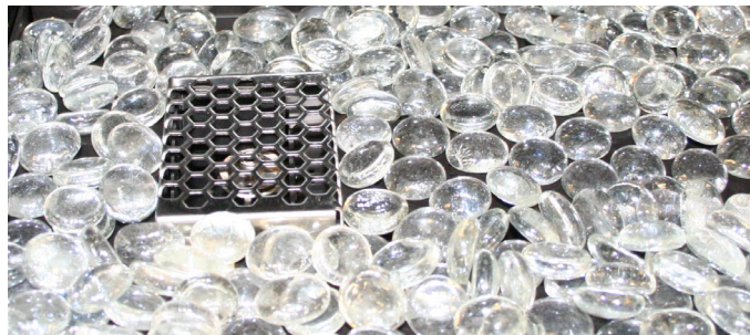
Figure 14d Gas fireplace with firestones covering burner tray.
