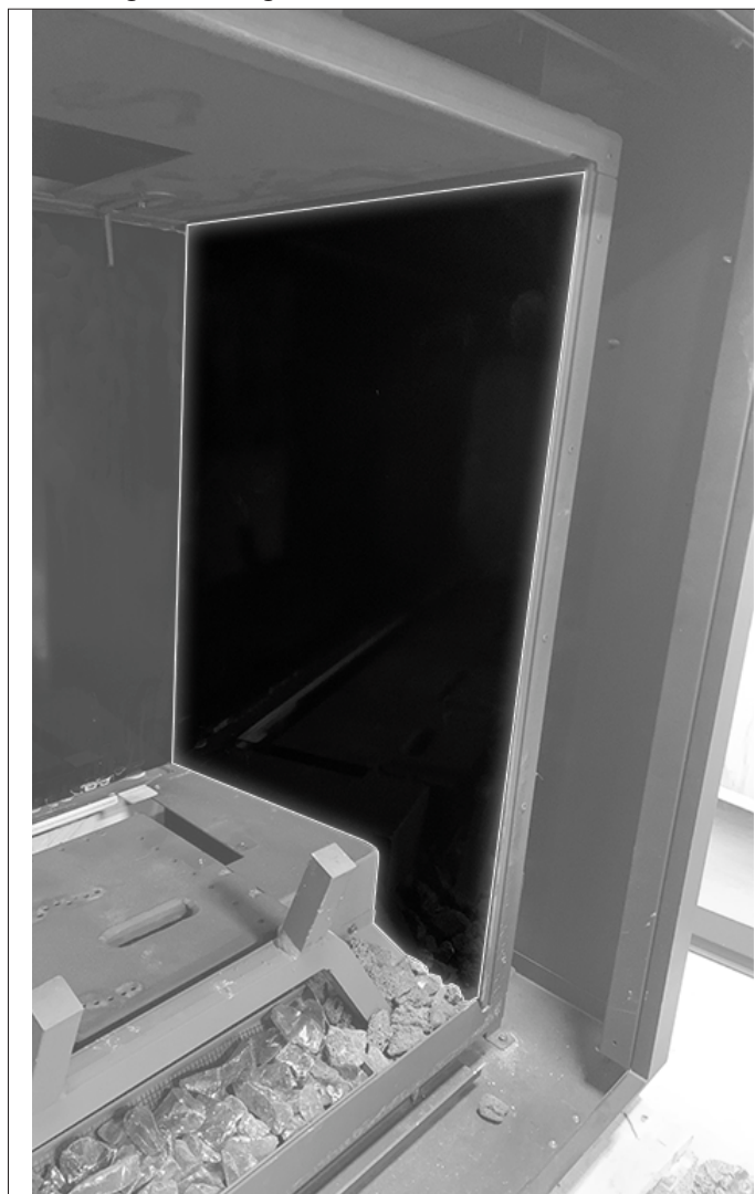
Figure 8.5, Side Black Glass Panels Installed
