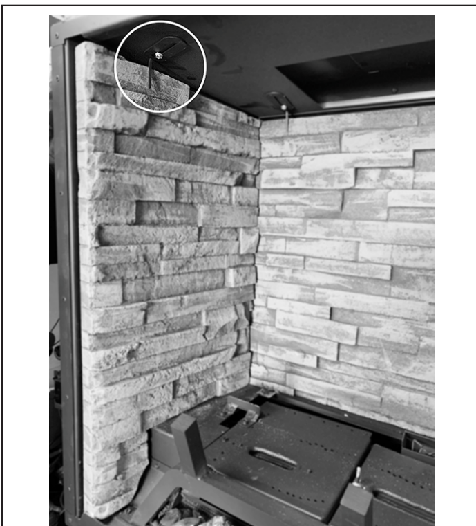
FIGURE 8.4 Side Refractory Panel Installed
