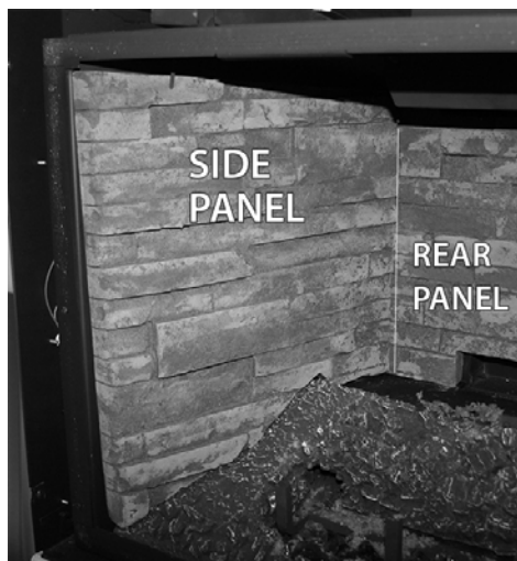
Figure 9.3, Refractory Panel Installation
