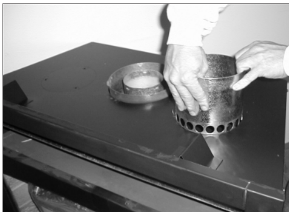
Figure 4.4, Duct Collar into Knockout
