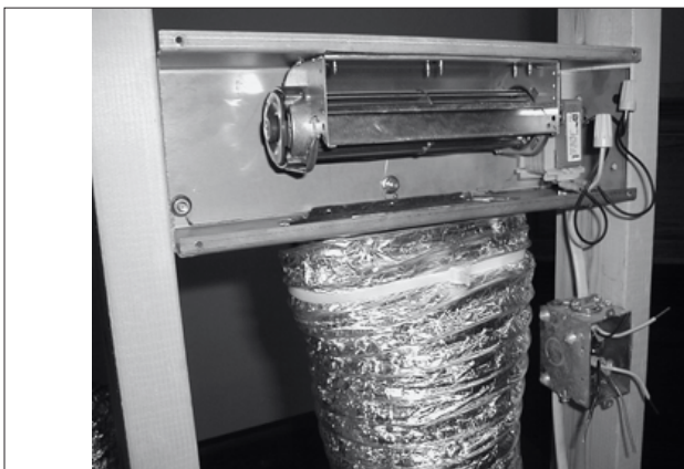
Figure 4.10, Secured Duct Pipe
