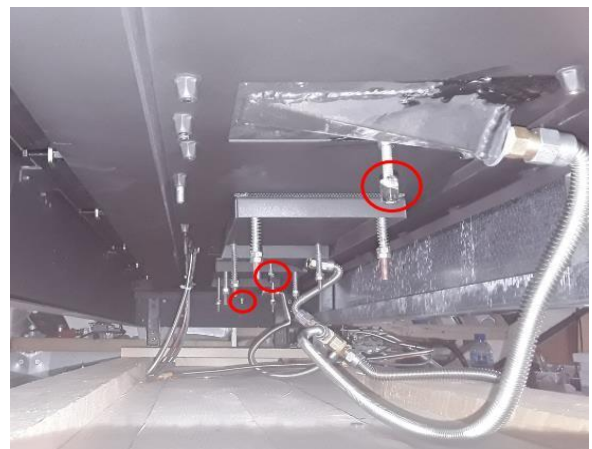
EX 2: AIR SHUTTER ADJUSTMENT UNDER YOUR FIREPLACE
