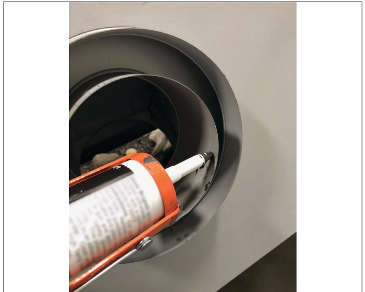
Figure 2.2, Joint scellant (silicone) au raccord d'évacuation interne du foyer
