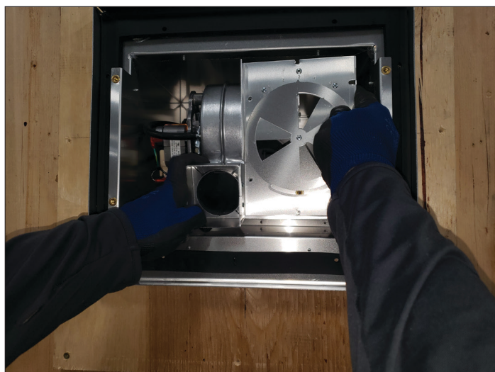
Figure 5.3, Exhaust Assembly Removal
