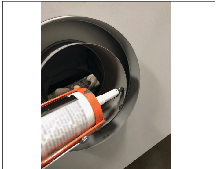
Figure 2.2, Silicone Inner Exhaust on Fireplace
