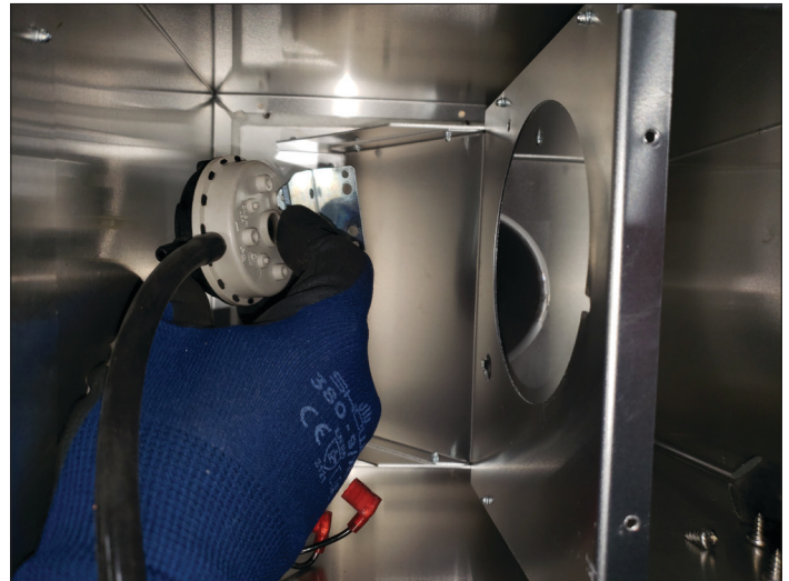
Figure 5.9, Vacuum Switch Removal
