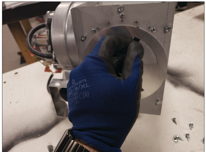
Figure 2.9, Adjust the Draft Bypass
