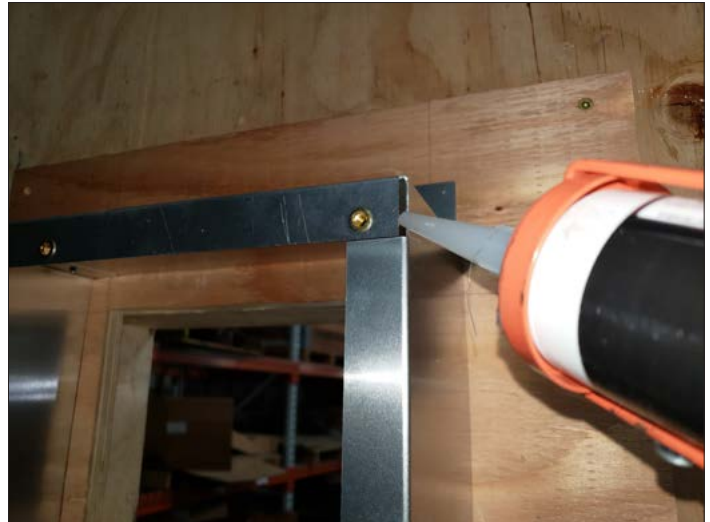
Figure 2.9, Appliquez le scellant silicone aux coins
